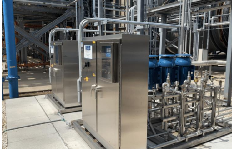
Figure 3. Typical Gas Turbine Inlet Fogging Skid (6)
