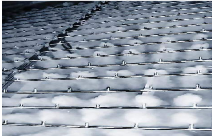
Figure (2): fog system in air intake gas turbine. [6]
